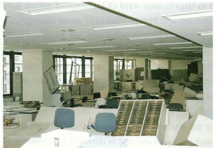
Photo. 3.2.1.48 Damage condition of the 7th roof floor of the 6th floor is pushed out to the 7th floor
