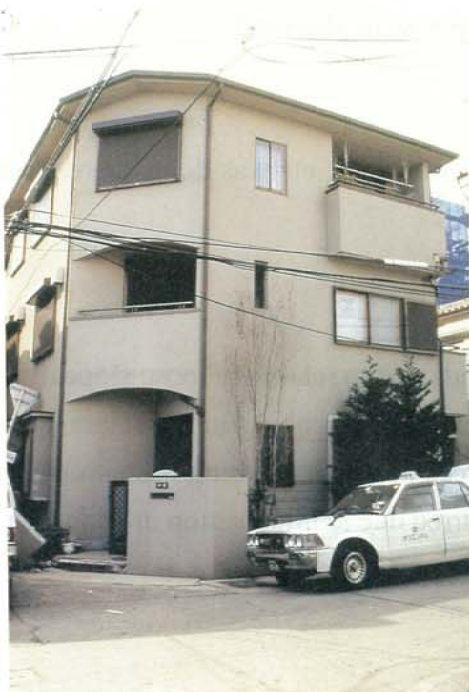
Photo 3.2.3.11 Three storey wooden building without damages
