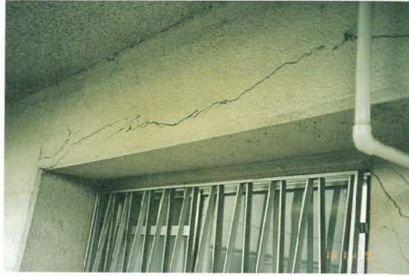
Photo.3.2.1.40 Bond splitting failure of a beam
