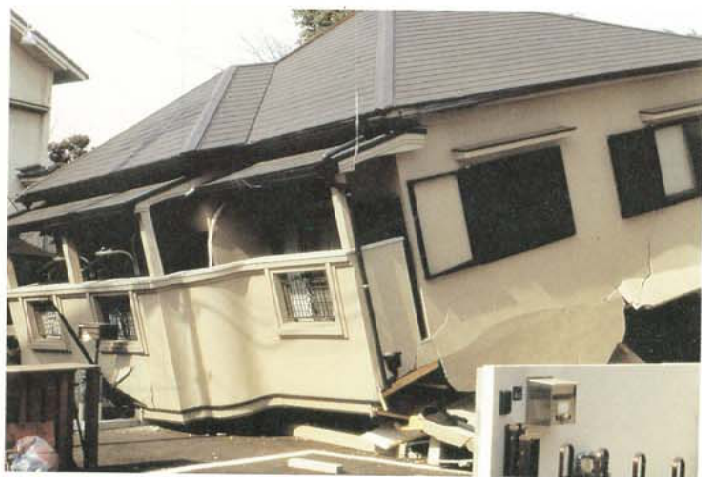
Photo 3.2.3.4 Collapse of the first story
