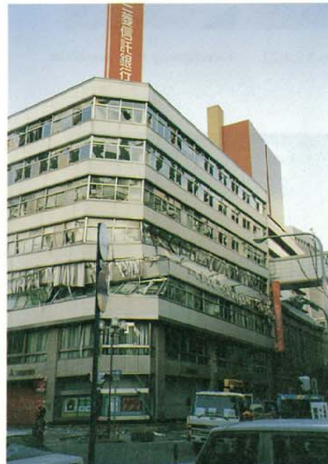
Photo. 3.2.1.19 Story collapse caused by the twist response
