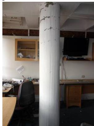
Photo 24-3 Bending-shear cracks of circular column
