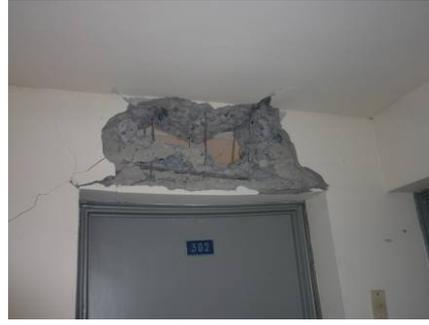
Photo 20-3 Shear failure of bearing walls and short span beam
