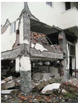
Photo 43-3 Failure of beam-column joint (Sichuan Earthquake, China, 2008)
