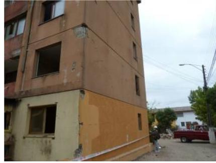
Photo 21-3 Damaged corner columns
