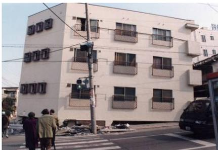
Photo 36-3 Collapse of soft first story structure
