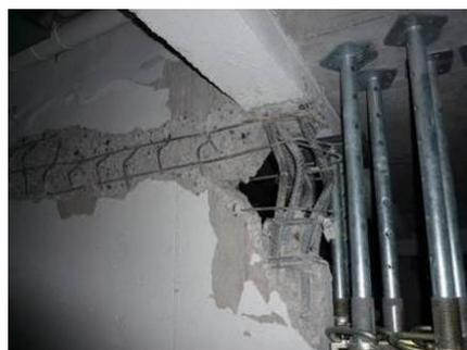
Photo 39-2 Smashed RC wall (Photo 2-3 reprinted)
