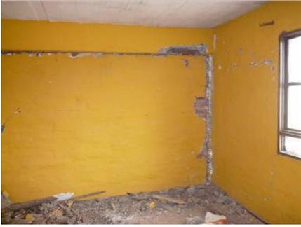
Photo 21-2 Damaged masonry wall
