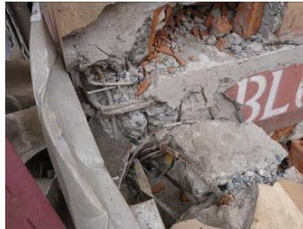
Photo 43-2 Failure of beam-column joint (Photo 14-4 reprinted)
