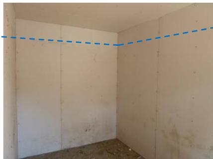
Photo 27-3 Trace of Tsunami (Wall at the second floor)
