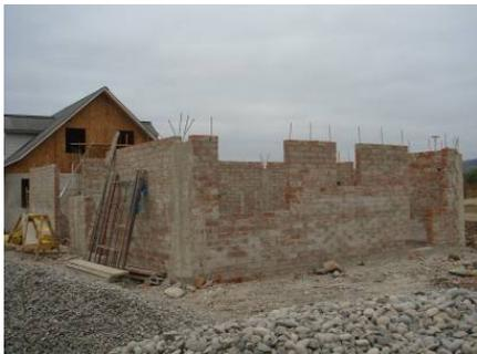
Photo 18-1 CM structure house under construction
