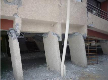
Photo 40-1 Flexural hinges on wall columns
