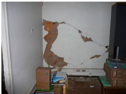
Photo 24-2 Damage of masonry e wall
