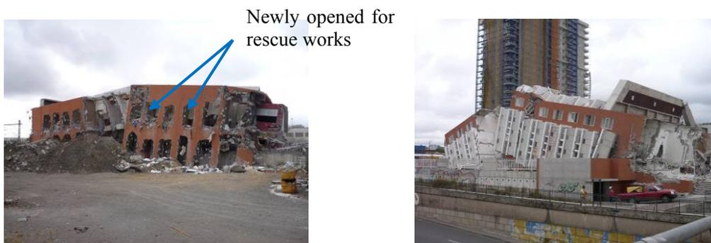
Photo 34-1 Damage of collapse (Photo 25-1 reprinted)
