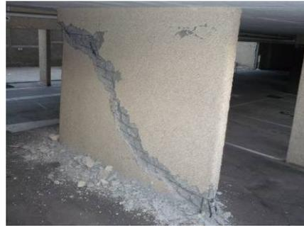
Photo 9-4 Shear failure
