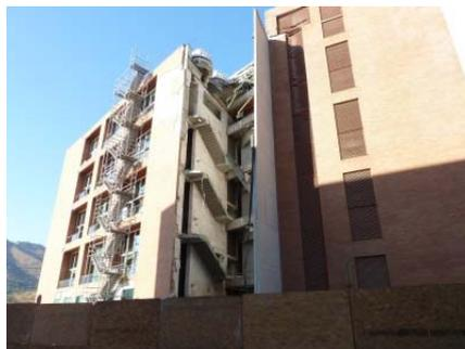
Photo 7-1 Appearance (crumbled external staircase)
