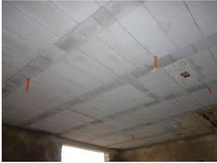
Photo 18-3 Joist slab
