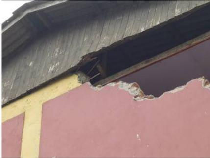
Photo 42-1 Failed beam at the top of the transverse wall (Photo 15-3 reprinted)
