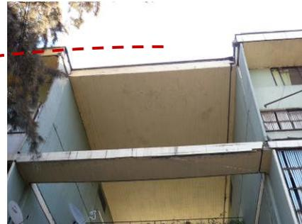
Photo 12-5 Fallen beam from roof
