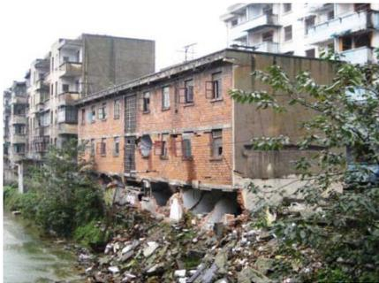
Photo 38-3 First floor collapsed brick construction building (Sichuan Earthquake, China, 2008)
