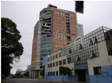
Photo 35-1 Collapse of the intermediate story (Photo 23-1 reprinted)
