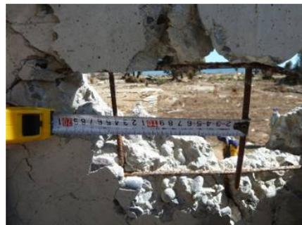
Photo 27-2 Precast RC construction
