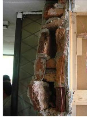
Photo 12-3 Damages of masonry walls
