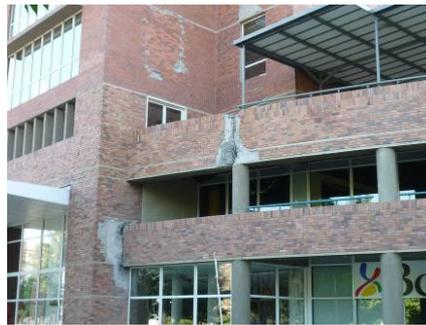
Photo 6-2 Damaged wall beam
