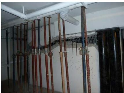
Photo 39-1 Smashed RC wall (Photo 1-2 reprinted)
