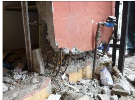
Photo 15-2 Shear failure of transverse wall
