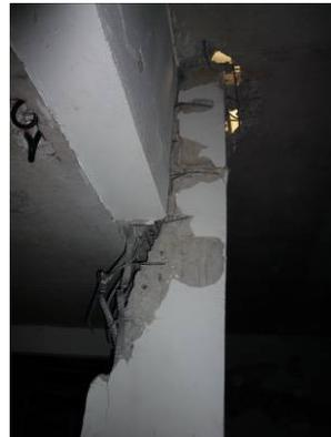
Photo 2-4 Damaged RC column
