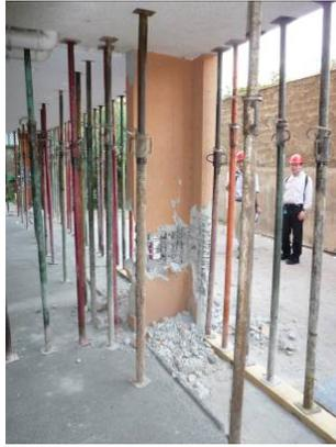
Photo 10-2 Damaged T-shaped wall columns and bearing walls
