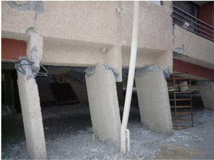
Photo 9-3 Wall column with bended hinge
