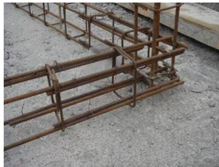
Photo 18-2 Bar arrangement of footing beam and corner
