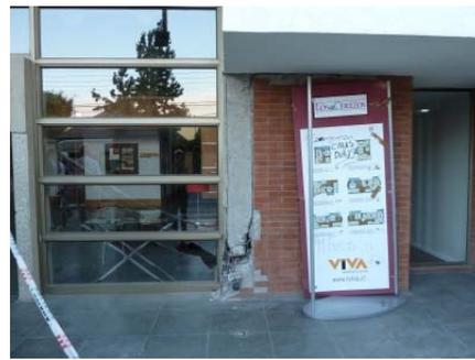
Photo 4-2 Crushed column bottom
