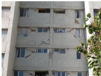
Photo 45-1 Cracks on brick walls (Photo 5-2 reprinted)
