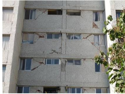
Photo 5-2 Damaged outer wall with bricks
