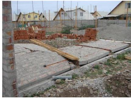
Photo 18-4 Fallen Masonry walls
