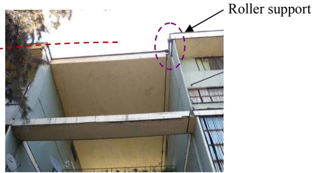
Photo 46-1 Drop of beam (Photo 12-5 reprinted)
