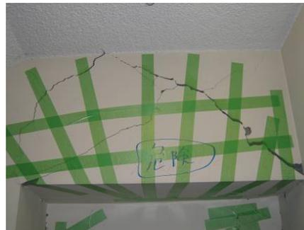
Photo 41-2 Shear cracks of short spanned
