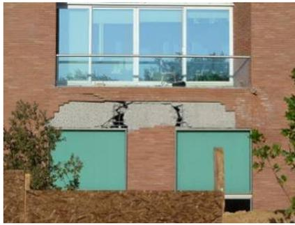
Photo 7-2 Damage on beam and beam-column joint
