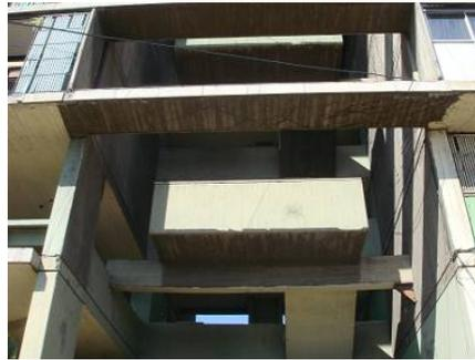
Photo 12-4 Cracks and deflection of beam at external staircase landing
