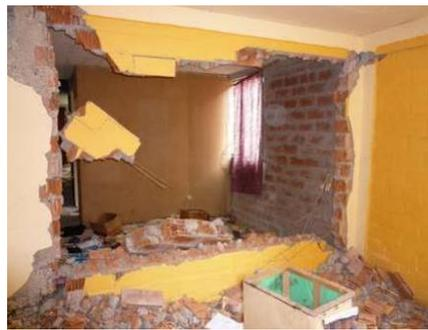
Photo 14-2 Columns and walls with CM structure
