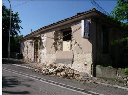
Photo 38-4 Masonry structure (L'Aquila Earthquake, Italy, 2009)
