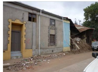
Photo 16-1 Damages of old brick structure and Adobe structure
