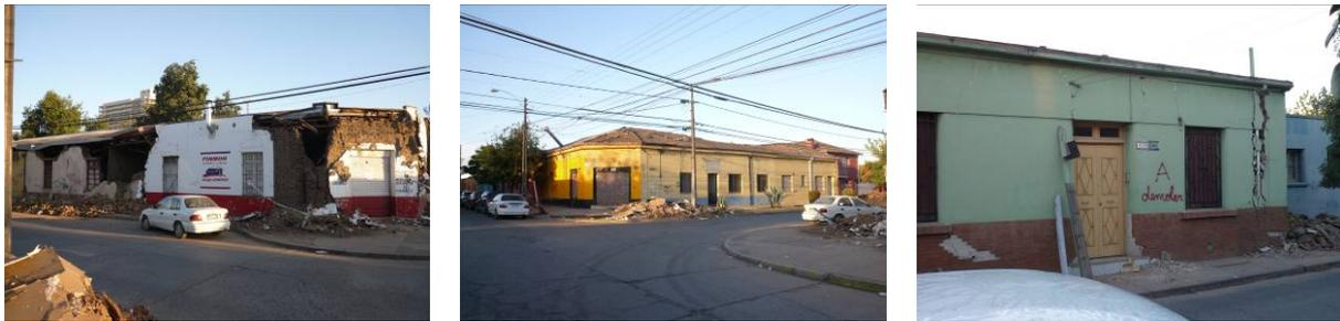
Photo 22-1 Damages of brick and adobe structures
