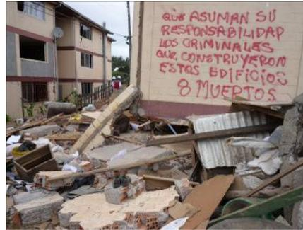
Photo 37-1 Collapsed first story of CM building (Photo 14-3 reprinted)
