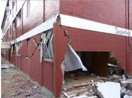
Photo17-1 Damaged transverse wall and longitudinal direction wall
