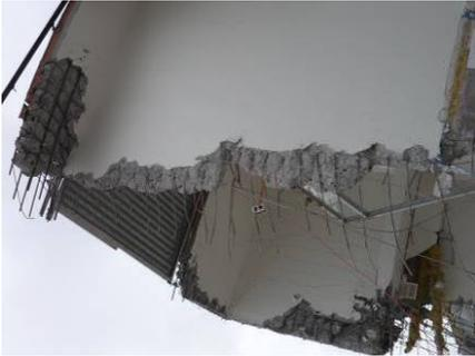
Photo 25-2 Torn wall columns and bearing walls
