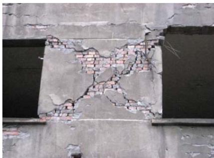
Photo 45-2 Collapse of nonstructural wall
