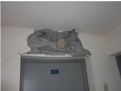
Photo 41-1 Shear failure of short spanned
