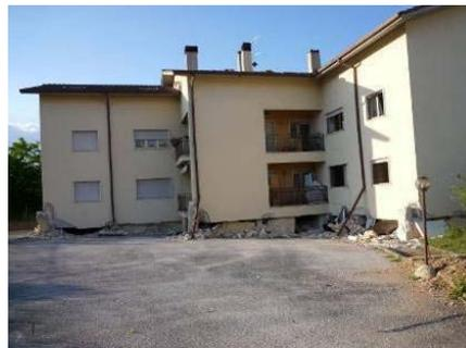
Photo 36-4 Collapse of soft first story structure
