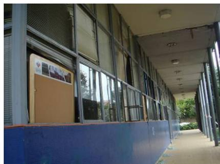
Photo 20-2 Longitudinal direction outer and broken windows
