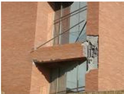
Photo 43-1 Failure of beam-column joint (Photo 7-2 reprinted)
