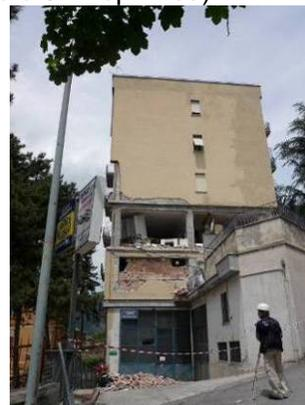
Photo 45-3 Collapse of brick walls
