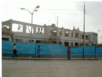
Photo 37-3 Collapsed CM buildings (Pisco Earthquake, Peru, 2007)
