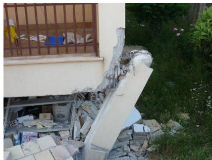
Photo 43-4 Failure of beam-column joint (L'Aquila Earthquake, Italy, 2009)
