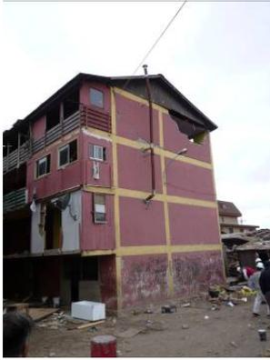
Photo 15-3 Damaged beam for top of transverse wall
