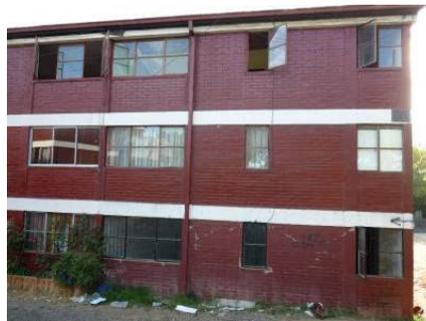
Photo 17-2 Shear cracks of longitudinal direction wall (Another building)
