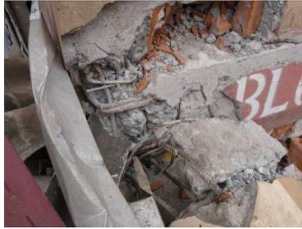
Photo 14-4 Beam-column joint
