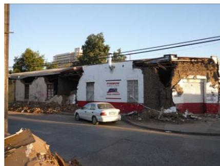
Photo 38-1 Damage of Adobe buildings (Photo 16-1, Photo 22-1 reprinted)
