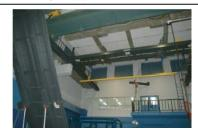
This baton can suspend a load up to 1 ton.
