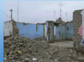
Collapsed adobe house (Nuevo Monterrico, Canete)
