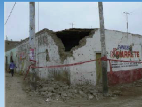
Adobe house with plaster spalling and corner destruction (San Luis, Canete)
