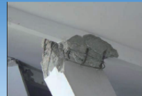
Close-up View of beam-column joint
