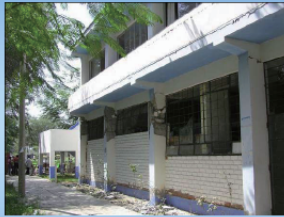
shear failure of short column with spandrel wall
