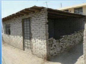
Collapsed adobe house (Nuevo Monterrico, Canete)
