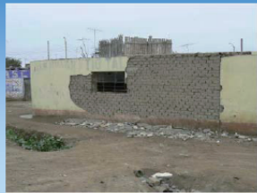
Adobe house with plaster spalling and corner destruction (San Luis, Canete)
