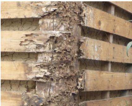
Photo 3.13 Bio-deterioration of Column and Based Mortar
