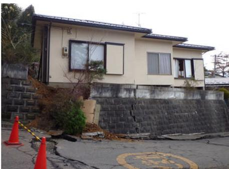
Photo 3.8 Damage of Retaining Wall and Houses (Oritate, Aoba Ward)
