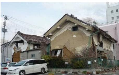
Photo 3.14 Dozo with Residual Deformation
