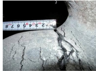
Photo 3.77 Lead Damper and Crack on the Surface
