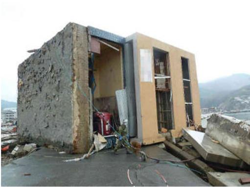
Photo 4.2 Overturning of 3-story Reinforced Concrete Building
