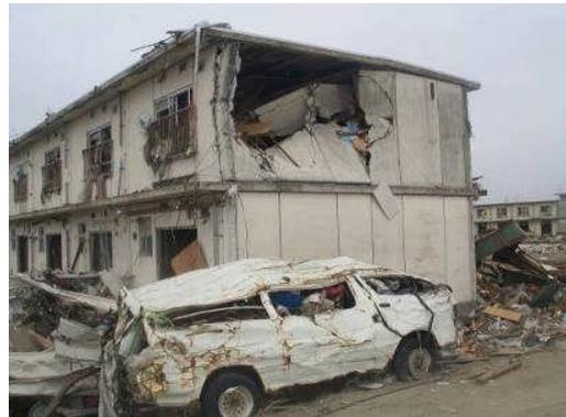
Photo 4.6 Wall Opening Generated by Debris Impact
