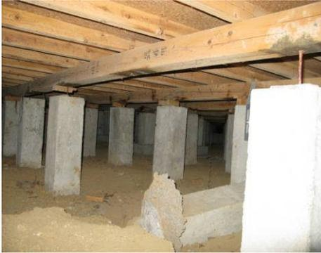
Photo 3.55 Overturning of Floor Strut
