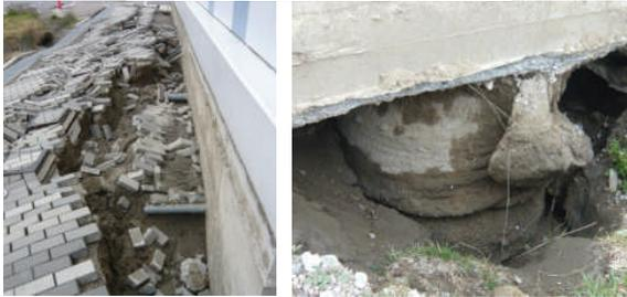
Photo 3.61 Situations around the Commercial Building and State of Pile Head
