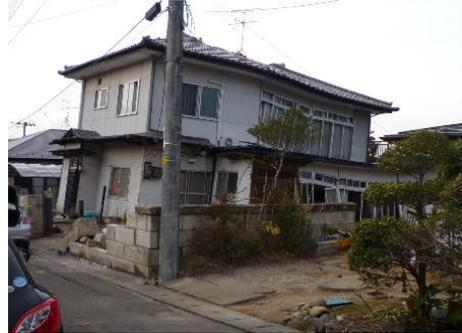
Photo 3.10 Damage of House caused by the Ground Transformation (Oritate)
