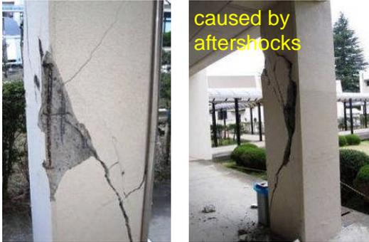
Photo 3.25 Shear Cracks on First-story Columns
