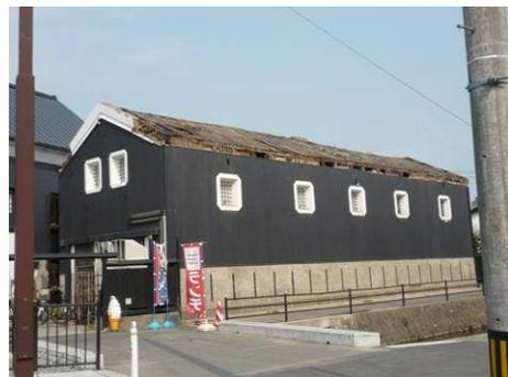
Photo 3.5 Warehouse with Mud Walls whose Roof System with Roof Tiles fell down
