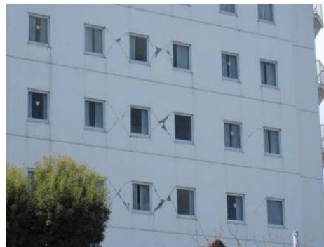
Photo 3.42 Shear Crack on Nonstructural Wall
