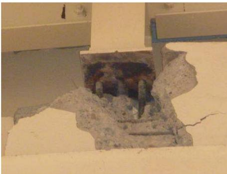
Photo 3.52 Spalling of Concrete
