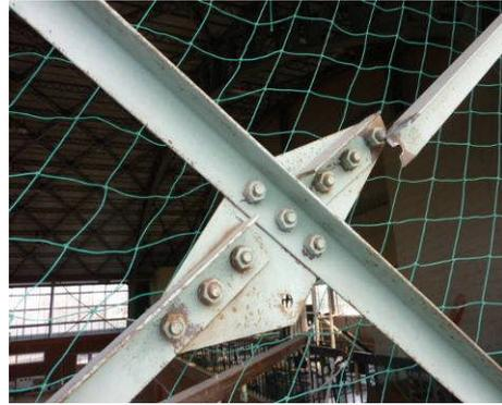
Photo 3.48 Net Section Fracture at Bolt Hole
