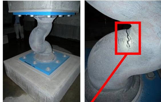
Photo 3.77 Lead Damper and Crack on the Surface
