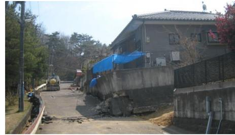
Photo 3.67 Damage of Retaining Wall and House Movement and Tilting by Sliding and Ground Transformation
