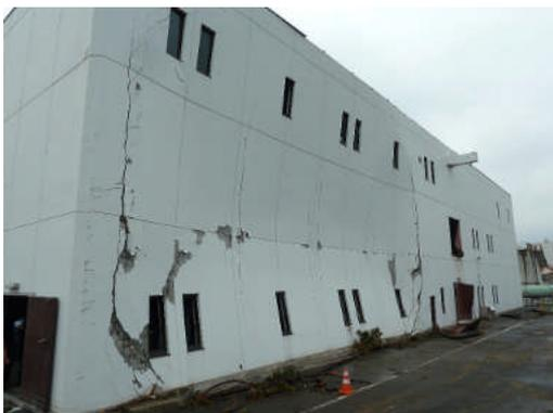
Photo 4.5 Out-of-plane Fracture of Reinforced Concrete Shear Wall without Floor
