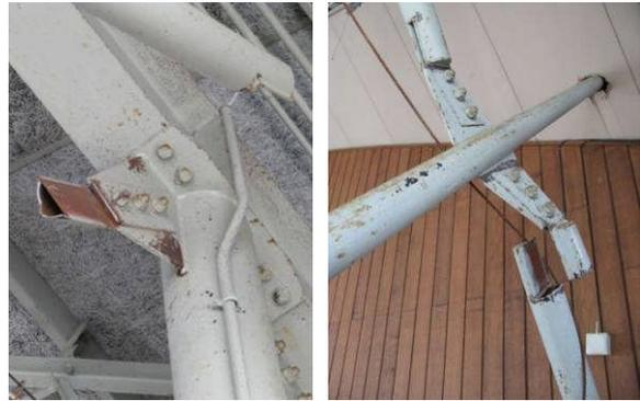
a) Fracture at column top b) Fracture at brace crossing
