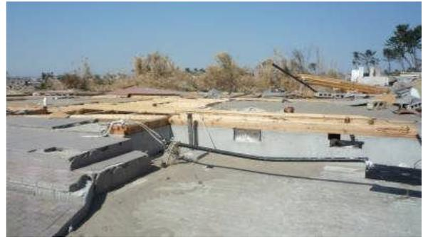
Photo 4.13 Remaining Ground Sill after Washout of Superstructure
