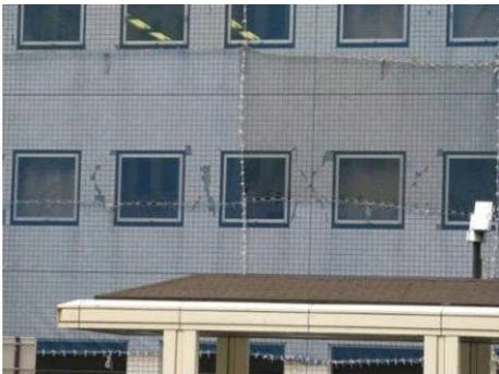
Photo 3.44 Damage of Tile on Exterior Wall
