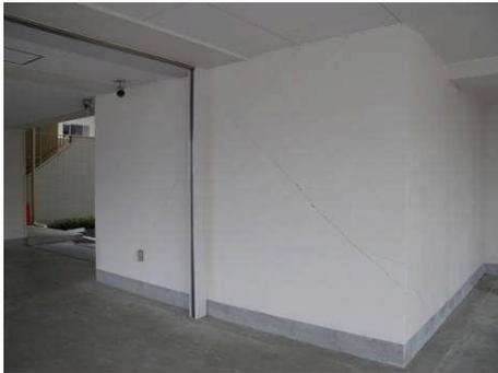
Photo 3.74 Shear Crack on the Wall
