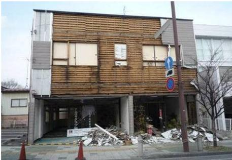
Photo 3.12 Fallen Mortar of Wall (Wood House with Shop)
