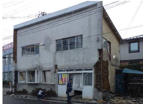
Photo 3.11 Drop Off the Mortar Wall (Komatsujima)
