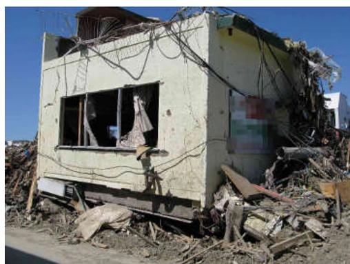
Photo 4.1 Story Collapse of 2-story Reinforced Concrete Building
