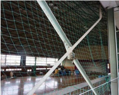
Photo 3.47 Buckling of Brace
