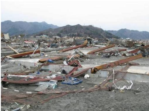
Photo 4.8 First-floor Columns Falling in the Same Direction
