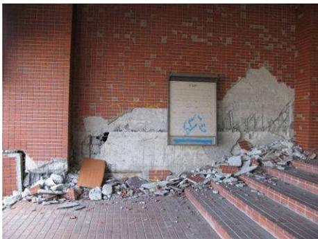
Photo 3.30 Damage on the Bottom of SRC Column and Shear Wall
