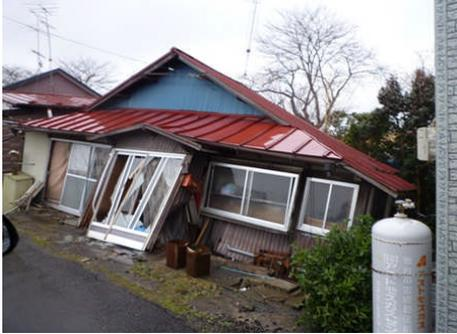
Photo 3.1 Damage of Houses caused by Ground Transformation
