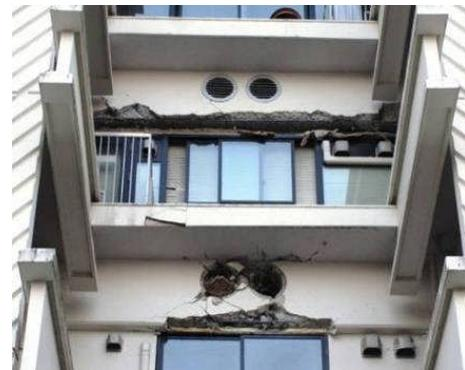
Photo 3.33 Damage on Boundary Beam with Opening
