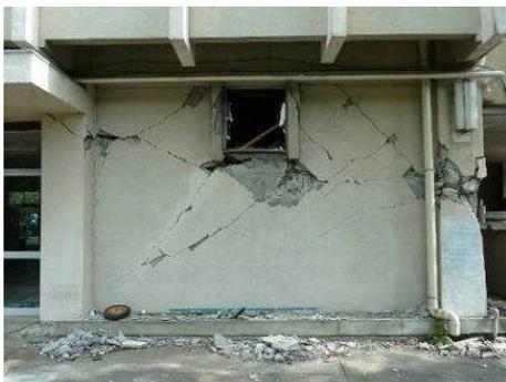
Photo 3.27 Shear Failure of Wall with Opening
