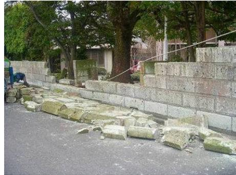
Photo 3.46 Collapse of Stone Masonry Wall
