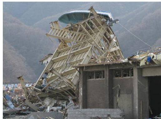
Photo 4.7 Steel Building Overturned by Fracture of Column Base Anchor Bolts
