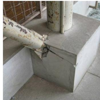
Photo 3.54 Cracking of Column Base Concrete
