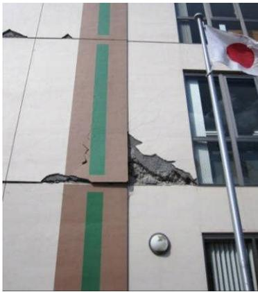
Photo 3.39 Separation of Concrete of Wing Wall
