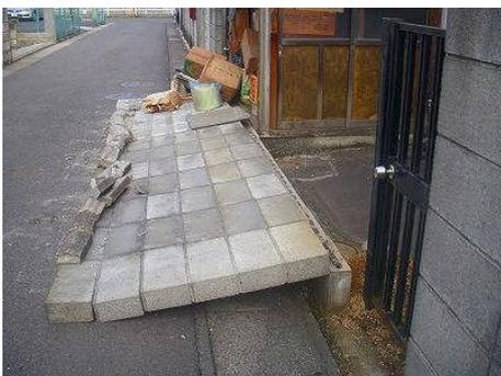
Photo 3.45 Collapse of Concrete Block Wall
