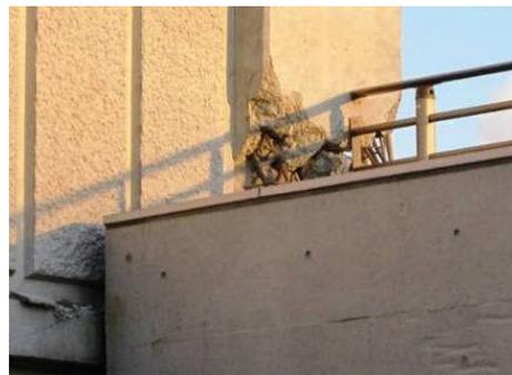
Photo 3.29 Crushing at the Bottom of Column on the Multi-story Shear Wall
