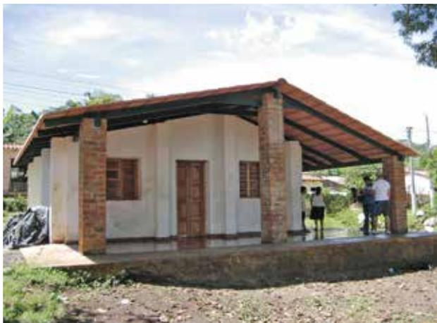
A model home built using the improved adobe construction method
