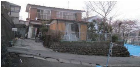
Photo 6.5-15 Damage to houses due to sliding and ground deformation
