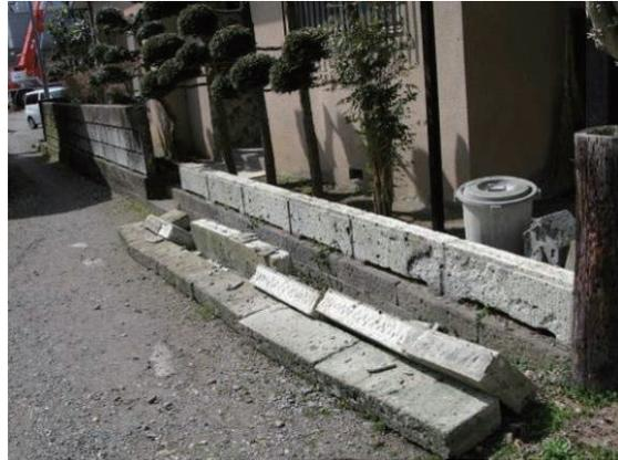
Photo 6.3-53 Collapse of stone masonry wall (Shirakawa city)
