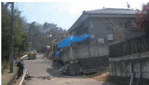
Photo 6.5-13 Damage to retaining wall and house due to sliding and ground deformation
