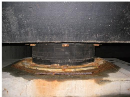
Photo 9.2-10 Rust of High-damping rubber bearing
