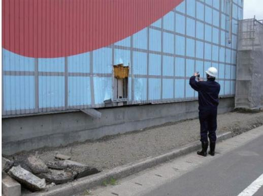
Photo 9.2-6 Damage due to debris
