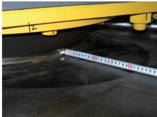
Photo 9.2-24 Trace of displacement of elastic sliding bearing
