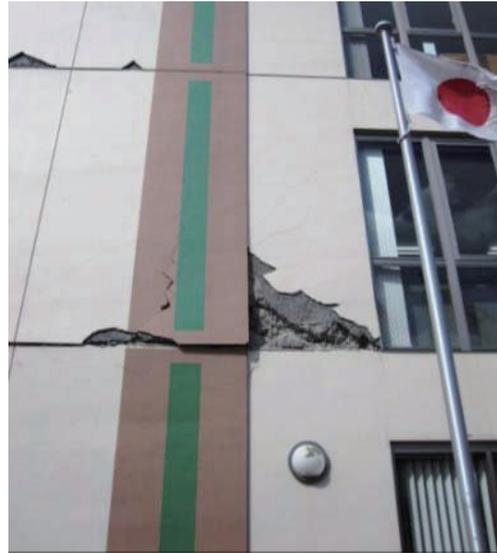
Photo 6.3-40 Separation of concrete of wing wall
