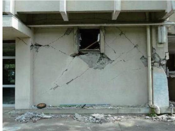
Photo 6.3-19 Shear failure of wall with opening
