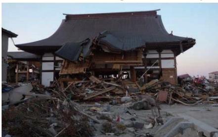
Photo 7.4-12. Heavily damaged temple (<sup>3</sup>) building in Yuriage, Natori city.
