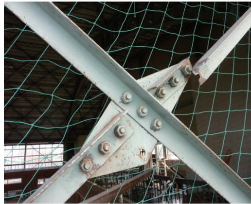
Photo 6.4-2 Net section fracture at bolt hole
