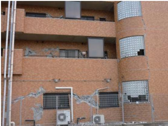
Photo 6.3-43 Damage of nonstructural wall in same building shown in Photo 6.3-22 (Koriyama city, Fukushima pref.)
