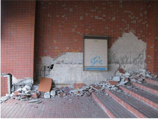
Photo 6.3-25 Damage of the bottom of SRC column and shear wall
