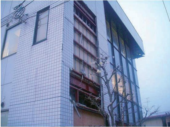
Photo 6.6-3 Falling of cement mortar and metal lath wall
