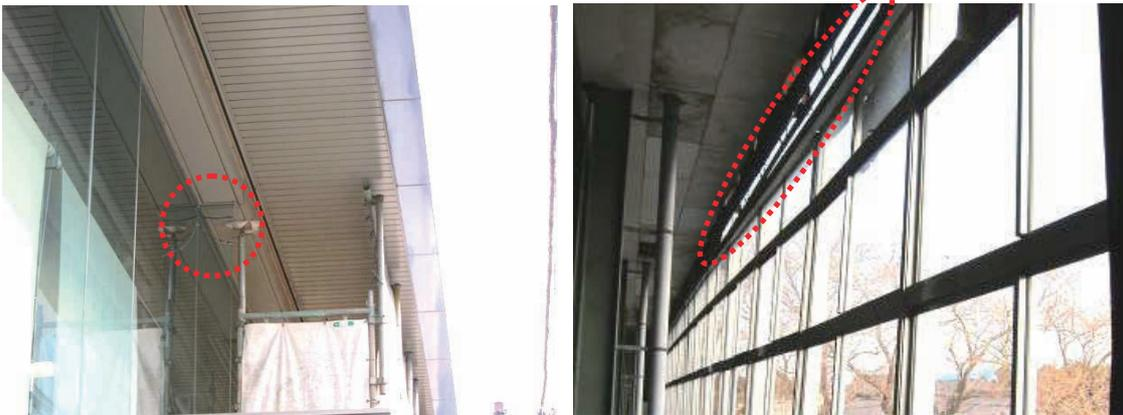
Photo 6.6-12 Breakage of glass mullion of glass wall system      Photo 6.6-13 Dislocation of window frame
