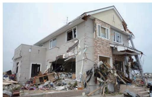
Photo 7.4-19. Light frame construction wood house (12) remained alone
