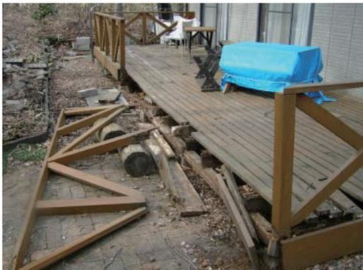
Photo 6.2-57 Damage of wood deck in Toyohara-Otsu, Nasu town
