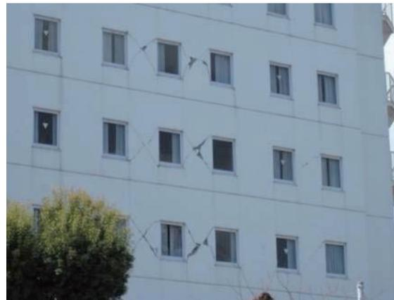
Photo 6.3-46 Shear crack on nonstructural wall
