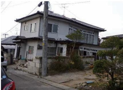
Photo 6.2-39 Damage of house caused by the ground transformation (Oritate)
