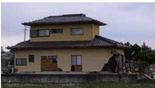
Photo 6.2-71 Falling down of mortar plastered wall
