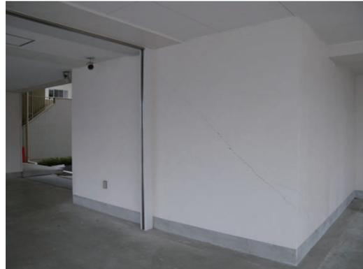
Photo 9.2-14 Shear crack on the wall
