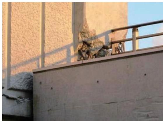
Photo 6.3-21 Crushing at the bottom of column of the multi-story shear wall
