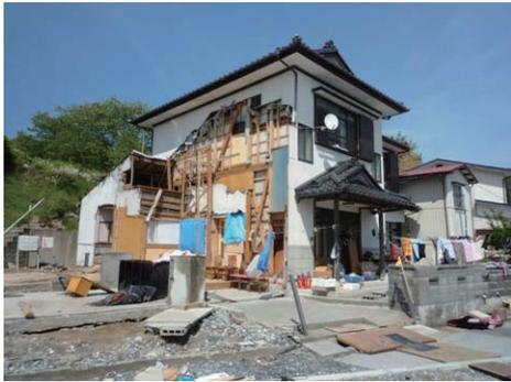
Photo 7.4-27. Wood house (11) remained under the water depth of over 7 m in Akasaki-cho, Oofunato city.
