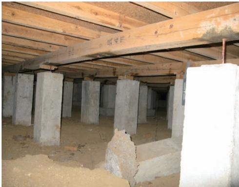
Photo 6.4-13 Overturning of floor strut
