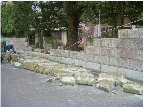
Photo 6.3-52 Collapse of stone masonry wall (Fukushima city)
