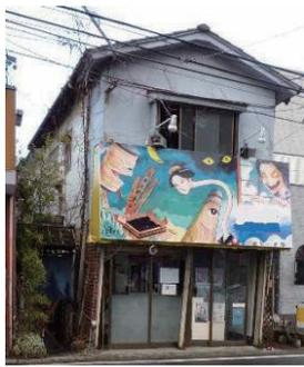
Photo 6.2-41 House with large residual deformation (Komatsujima)
