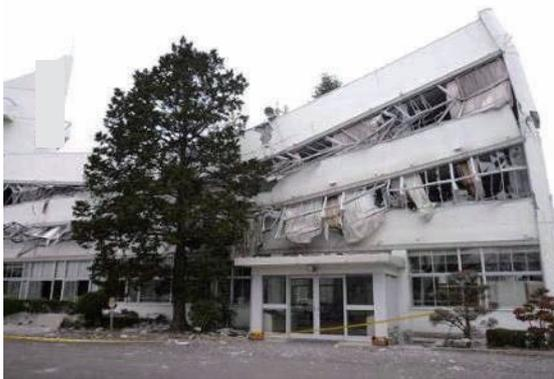
Photo 6.3-7 Mid-story collapsed building (Fukushima city)
