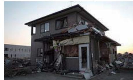
Photo 7.4-13. Wood house with store (<sup>5</sup>) remained in the downstream of the survived buildings in Yuriage.
