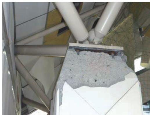
Photo 6.4-7 Spalling of concrete
