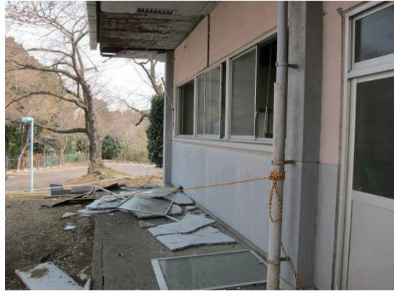
Photo 6.6-4 Falling of cement mortar and metal lath from eaves soffit
