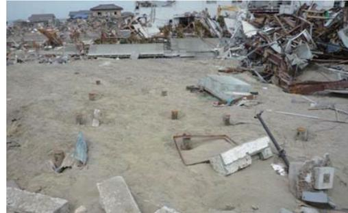
Photo 7.4-11. Steel tube pile left at the original position (<sup>2</sup>) of house in photo 7.4-10.
