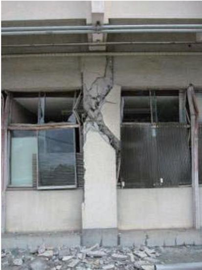
Photo 6.3-18 Shear failure of column
