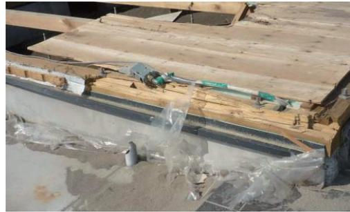
Photo.7.4-4. Sills, foundation and floor boards remained.
