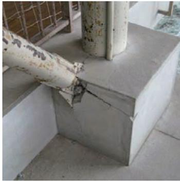
Photo 6.4-11 Cracking of column base concrete
