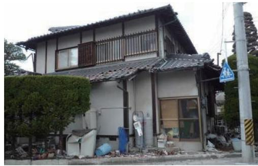
Photo 6.2-49 Damage of roof tile
