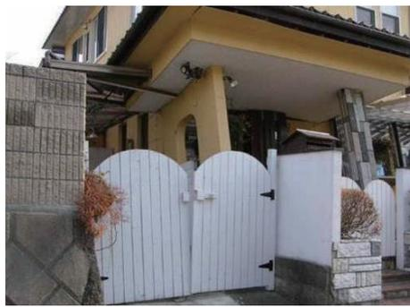
Photo 6.2-68 Wood house with large shear deformation
