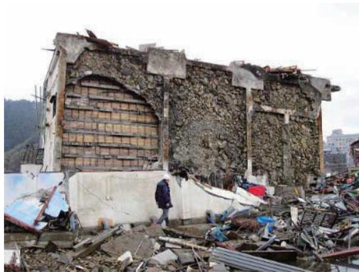
Photo 7.2-3 A 2-story reinforced concrete building that moved over the fence and overturned
