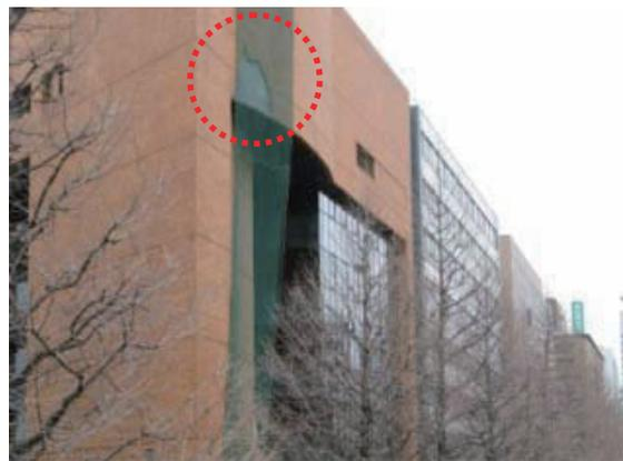
Photo 6.6-2 Detachment of ceramic wall tiles from RC wall
