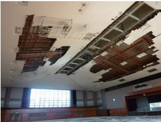
Photo 6.6-15 Falling of metal furring suspended ceiling
