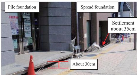
Photo 6.5-11 Difference in damage due to support mechanisms
