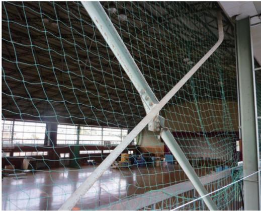
Photo 6.4-1 Buckling of brace
