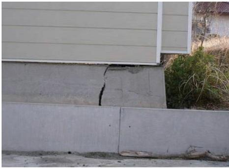
Photo 6.2-67 Crack of foundation
