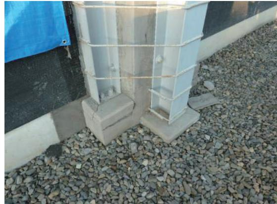
Photo 6.3-11 Column strengthened with H-shaped steel
