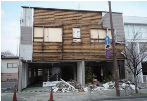
Photo 6.2-44 Fallen mortar of wall (Wood house with store)
