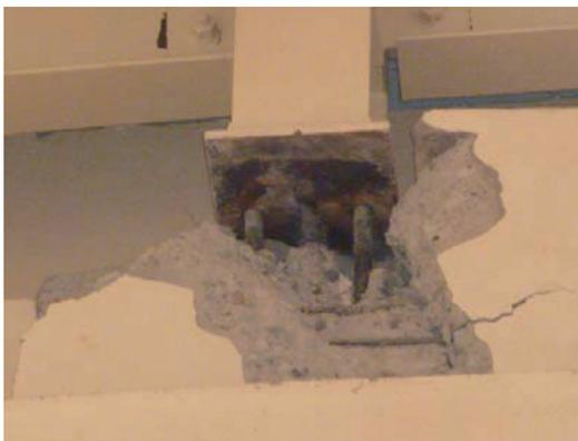
Photo 6.4-6 Spalling of concrete
