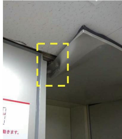
(b) Damage to the expansion joint
