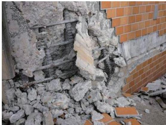
Photo 6.3-23 Damage at the bottom of SRC column
