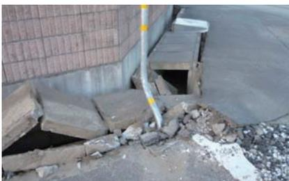
Photo 6.5-6 Damage to side ditch
