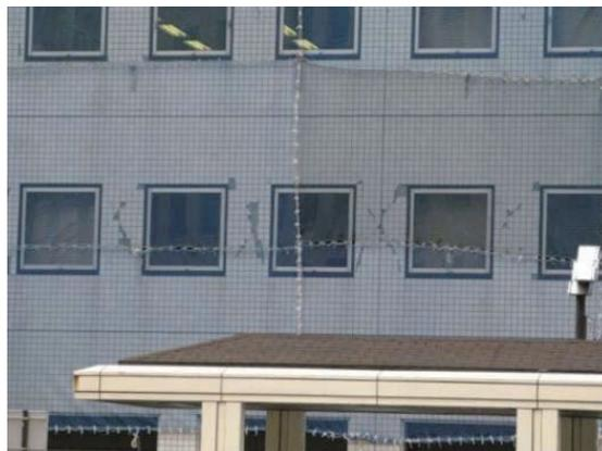
Photo 6.3-49 Damage of tile on exterior wall
