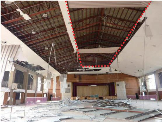
Photo 6.6-17 Falling of metal furring suspended ceiling and corrugated steel plates
