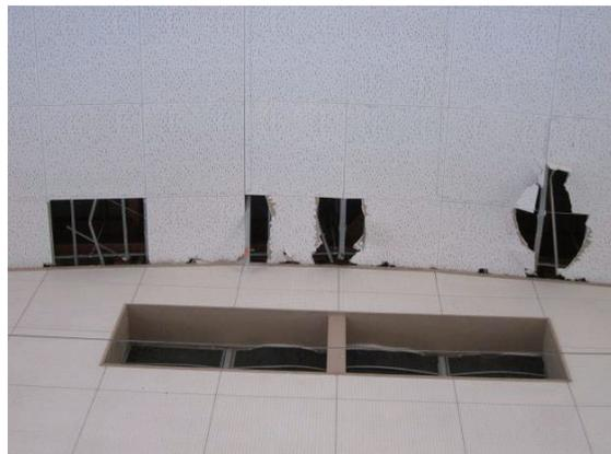
Photo 6.6-20 Damage to metal furring ceiling at the connection wall
