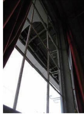
Photo 6.4-21 Falling of eave soffit
