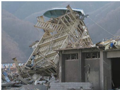
Photo 7.2-7 Steel building overturned by fracture of column base anchor bolts
