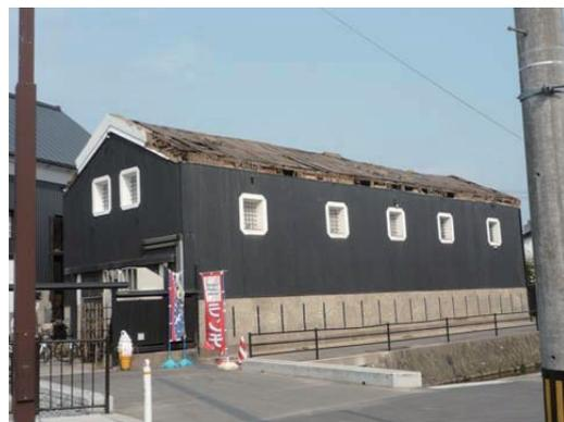
Photo 6.2-12 Warehouse with mud walls whose roof system with roof tiles fell down
