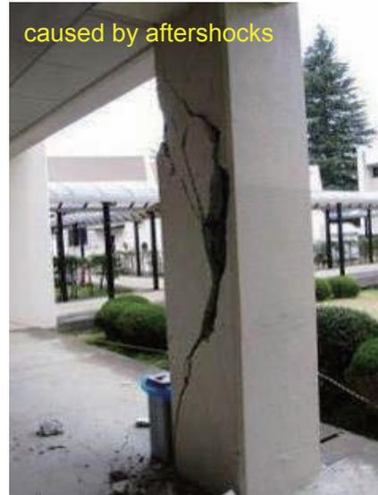
Photo 6.3-13 Shear cracks of first-story columns
