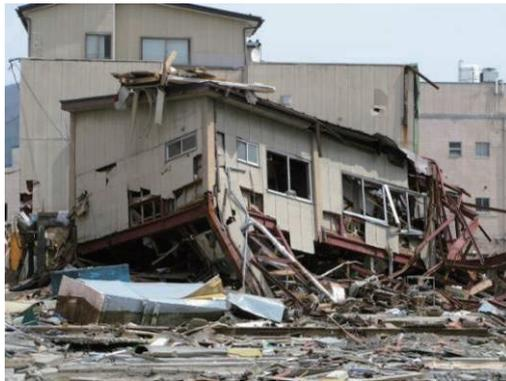
Photo 7.2-10 Story collapse of first floor in a 2-story steel building
