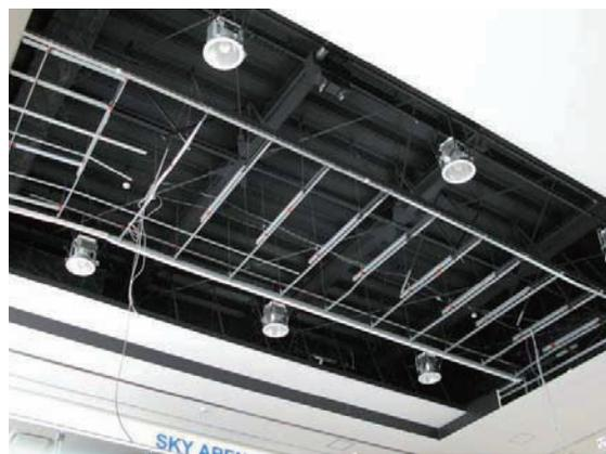
Photo 6.6-16 Falling of metal furring suspended ceiling
