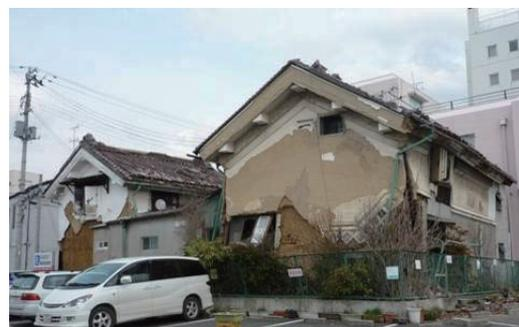
Photo 6.2-47 Failed warehouse with mud wall
