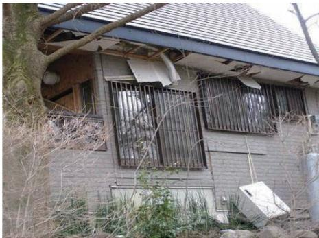
Photo 6.2-61 Failed ceiling of eave
