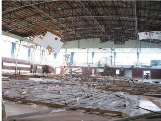
Photo 6.6-14 Falling of wooden suspended ceiling
