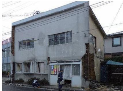
Photo 6.2-40 Drop off the mortar wall (Komatsujima)
