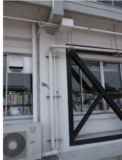
Photo 6.3-38 Shear crack on column with framed steel braces
