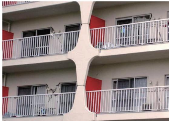
Photo 6.3-31 Shear cracks on mullion
