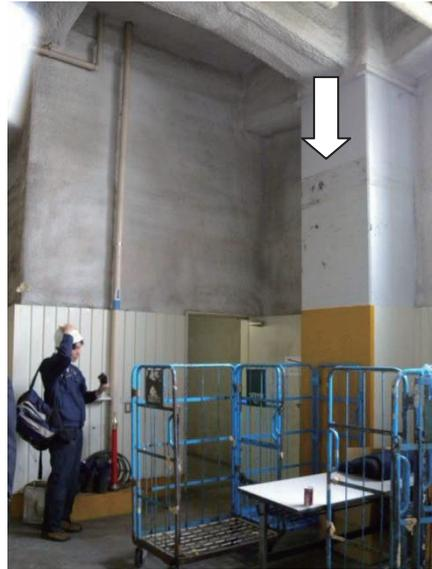
Photo 9.2-7 Trace of tsunami water
