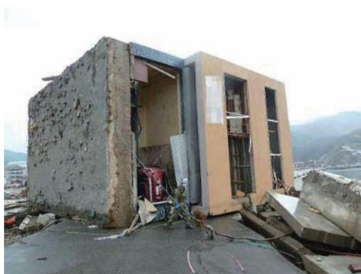
Photo 7.2-2 Overturning of a 3-story reinforced concrete building
