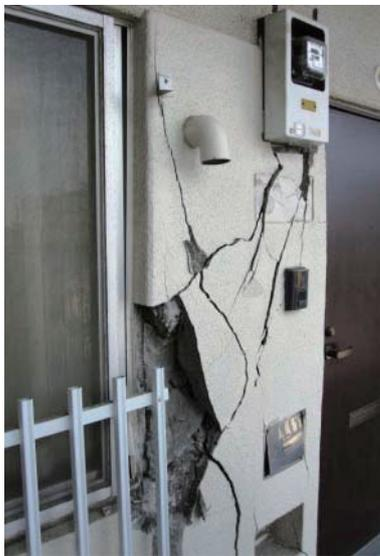
Photo 6.3-30 Shear cracks on nonstructural wall
