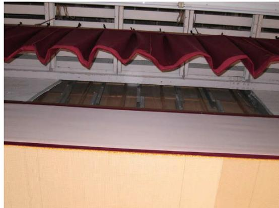
Photo 6.6-23 Falling of cement mortar finish above stage
