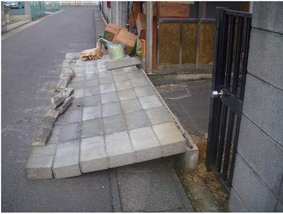
Photo 6.3-50 Collapse of concrete block wall (Koriyama city)
