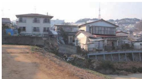
Photo 6.5-14 Group of houses damaged due to sliding and ground deformation
