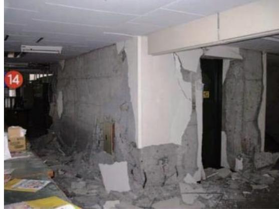
Photo 6.3-16 Failure of shear wall
