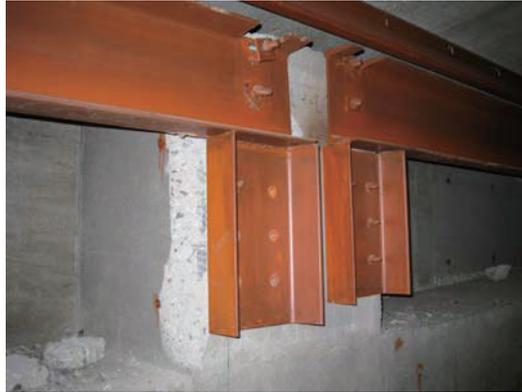
Photo 6.4-8 Pullout of hole-in anchors
