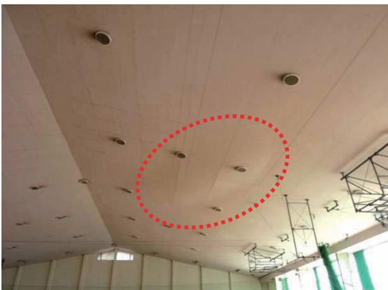
Photo 6.6-19 Sagging of metal furring suspended ceiling
