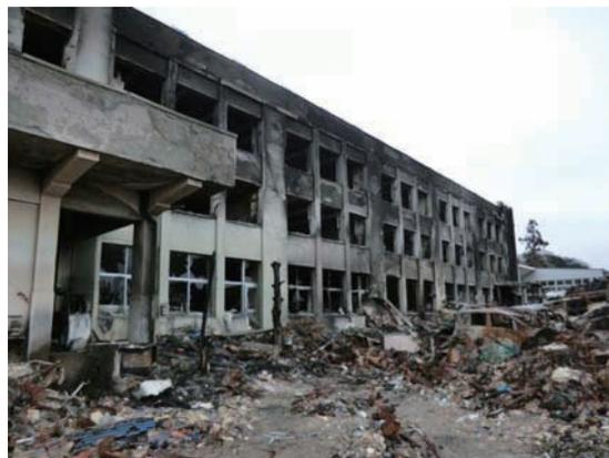
Photo 8.2-1 Tsunami fire at an elementary school (Ishinomaki city, Miyagi prefecture)
