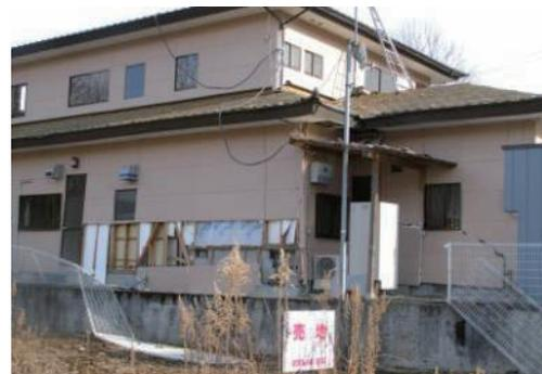
Photo 6.2-64 Damaged house due to deformation of residential land
