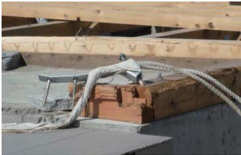
Photo.7.4-5. Failed hold down fastener.
