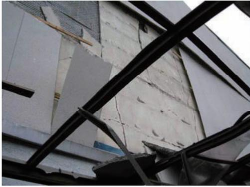
Photo 6.4-20 Falling of exterior finish components
