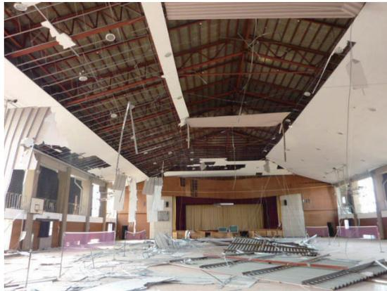
Photo 6.4-18 Dropping of extensive ceiling components
