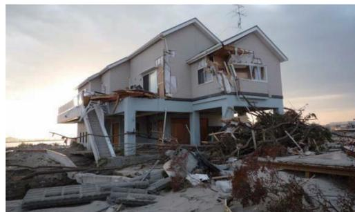
Photo 7.4-23. Mixed structure which has 1<sup>st</sup> story of RC structure and wooden 2<sup>nd</sup> story.
