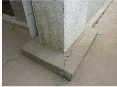
Photo 6.4-12 Cracking of column base concrete
