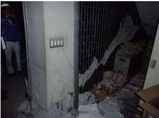
Photo 6.3-10 Shear crack on shear wall
