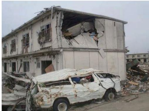
Photo 7.2-6 Wall opening probably generated by debris impact
