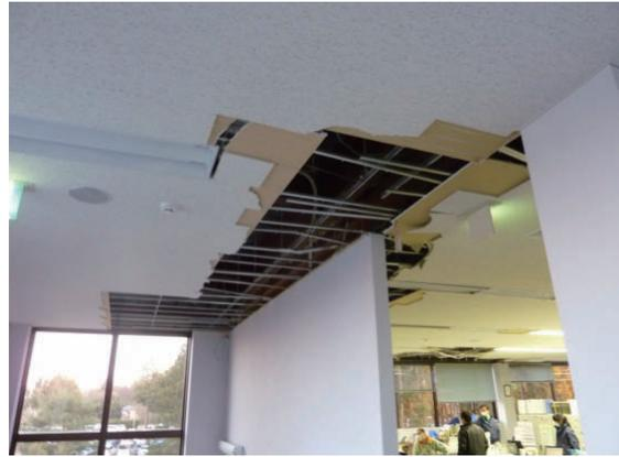
Photo 6.6-22 Damage to metal furring suspended ceiling at the connection
