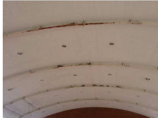
Photo 6.4-14 Peeling of paint of beams
