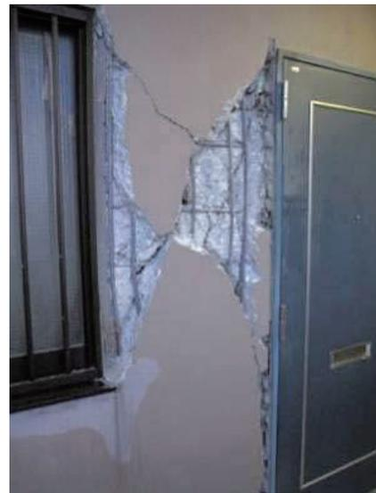
Photo 6.3-42 Shear failure of nonstructural wall
