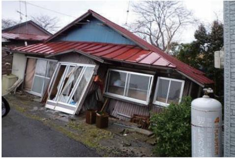
Photo 6.2-3 Damage of houses caused by ground transformation
