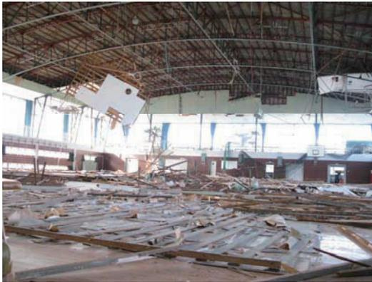
Photo 6.4-16 Dropping of extensive ceiling components
