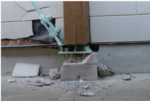
Photo 6.2-78 Breakage of the foundation concrete
