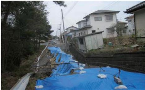
Photo 6.5-17 Fracture of embankment retaining wall and houses tilting due to land sliding on the slope of hill end
