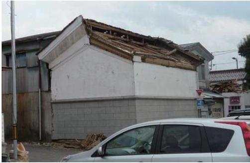
Photo 6.2-48 Fallen roof of warehouse with mud wall
