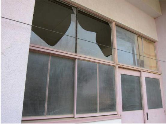
Photo 6.6-9 Breakage of window glasses installed to fixed window frame with hardening putty
