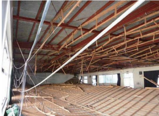
Photo 6.4-17 Dropping of extensive ceiling components
