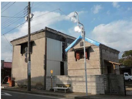
Photo 6.2-55 Damage of stone-built warehouses
