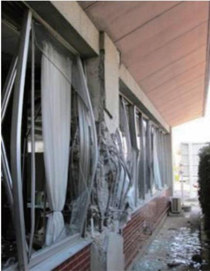
Photo 6.3-15 Shear failure of short column
