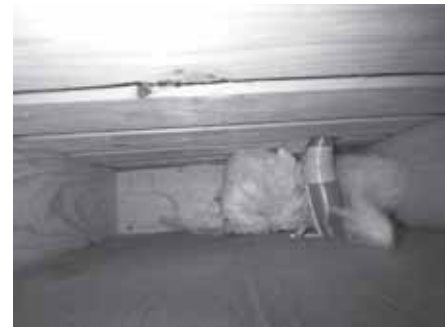
Fig. 4 Example of insulation being drilled with hole saw
