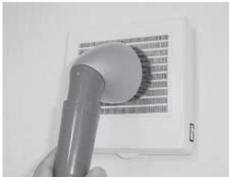
Fig. 12 Cleaning filter of through-the-wall exhaust fan
