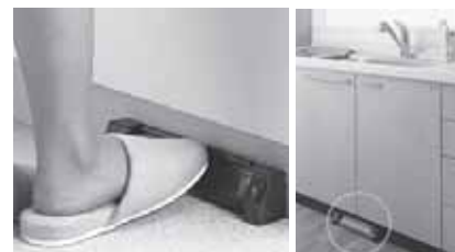
Fig. 19 Example of foot-controlled water shut off
